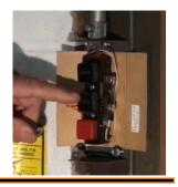
2. Install the new door switch/receiver to the same location on the wall. Install the wires to the 3 switches from which they were removed in Step 1.
